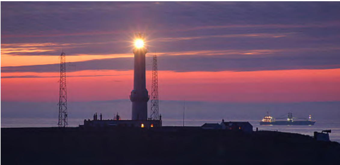
Girdle Ness Lighthouse - ONE OF THE UK DGPS REFERENCE STATIONS
