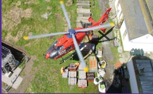
Pladda Lighthouse site clearance
